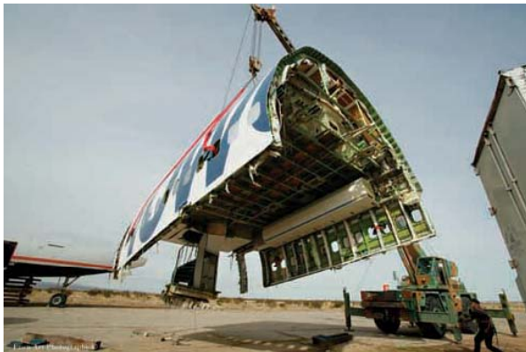
Deconstruction of Boeing 747 parts for future use in Wing House construction
